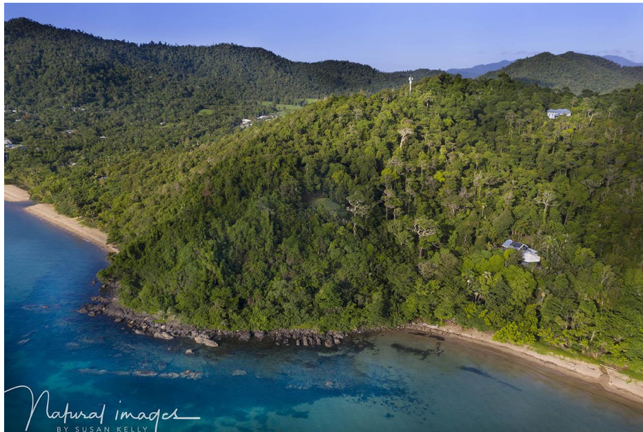
2021, Bingil Bay (left) and Brookes Beach (right) showing Sid Cutten's two beachfront lots, Lot 158 and Portion 19v (foreground). Image courtesy Susan Kelly, Natural Images .
