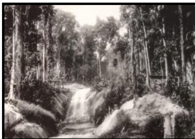
Road across Lacey's Creek before the bridge was erected, early 1930's.
