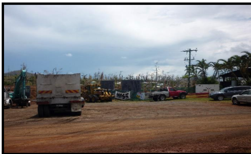
Construction commenced after Cyclone Yasi, March 2011
