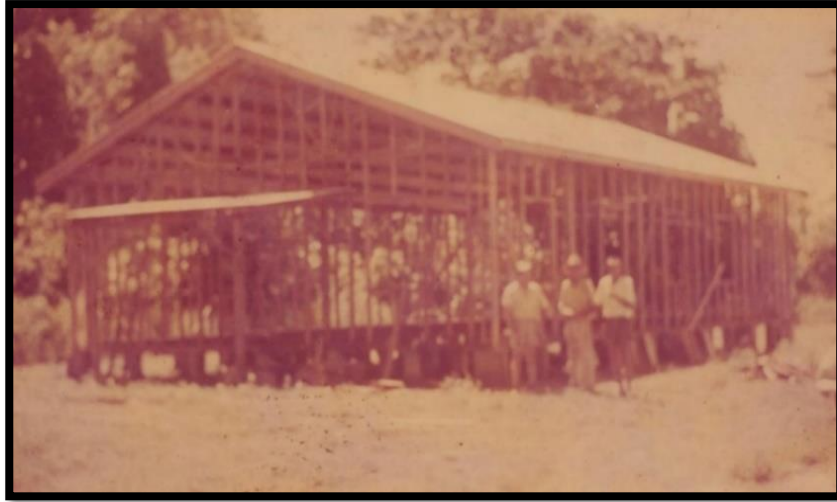
Building the Progress Hall, 1964.
