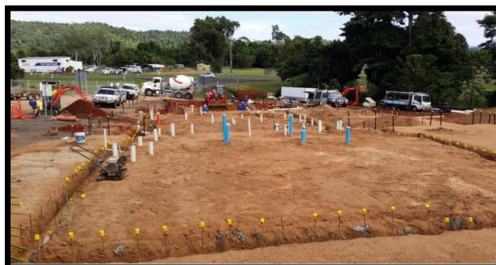
First concrete truck arrives, June 2017
