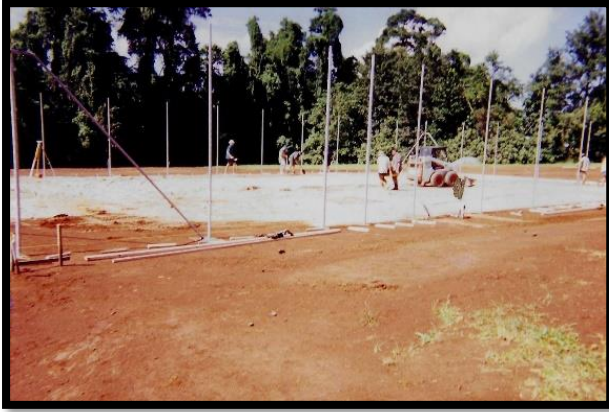
Construction of the courts, 2000.
