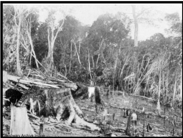
Clearing land for Hull River Aboriginal Settlement 1914
