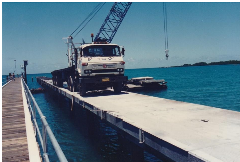
Removing the old 1963 concrete jetty – new timber one (third jetty) alongside, 1994.
