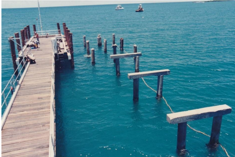
Second (concrete) jetty almost all gone, third (timber) built.
