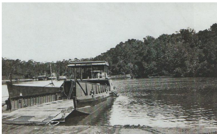
Barge at Markham River, Lae, 1953. From Doug Unsworth.
