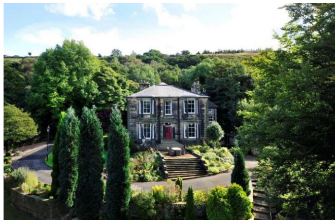
Cellars Clough House converted to units.
