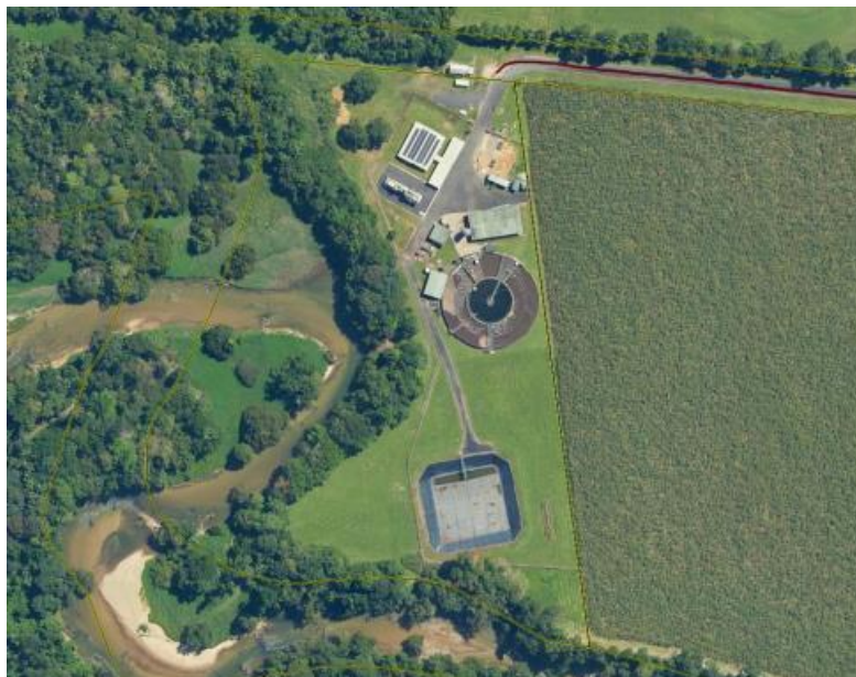
An aerial image shows Tully STP next to Banyan Creek. Image from CCRC Sewerage Report..
