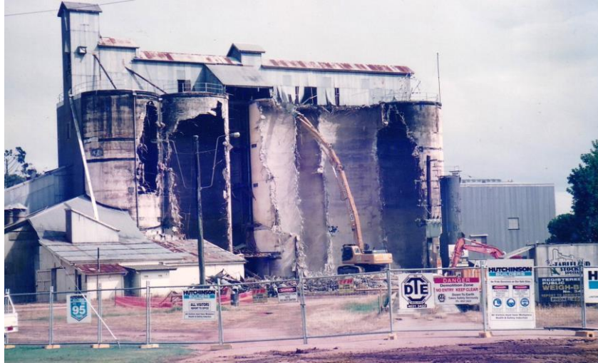
Atherton corn silos being demolished.
